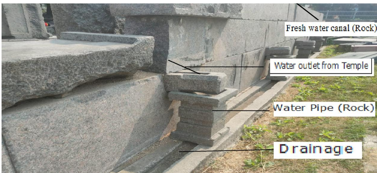
(Water flow.. in Shivalayam complex. Warangal Fort, Warangal)
